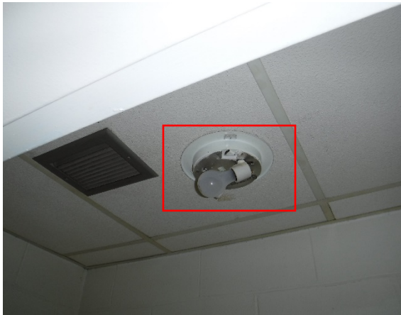
Photo 75: Photo of sample AS-34, Room 105, Bathroom – Lighting Unit Heat Shield, 45% Chrysotile Asbestos.
