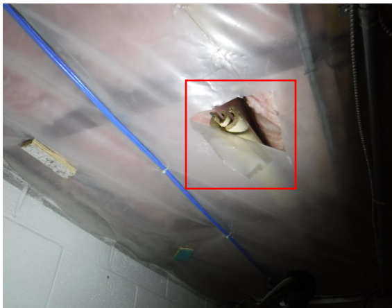
Photo 23: Example Photo of Poor Condition, Damaged ACM Piping Insulation, Straight Run – Room 118, Ceiling Cavity.
