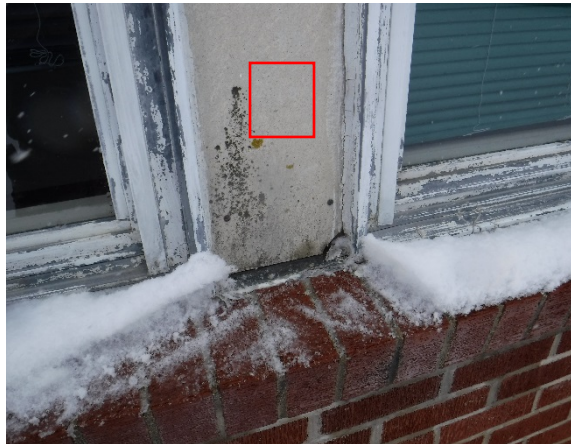
Photo 86: Photo of sample EXT-AS-01, Building Exterior – Transite Panel, 13.6% Chrysotile Asbestos.
