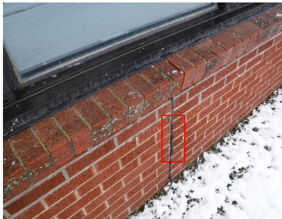
Photo 108: Photo of sample EXT-AS-03, Building Exterior, Wall – Expansion Joint Compound, Black/White, 0.76% - 1.2% Chrysotile Asbestos.
