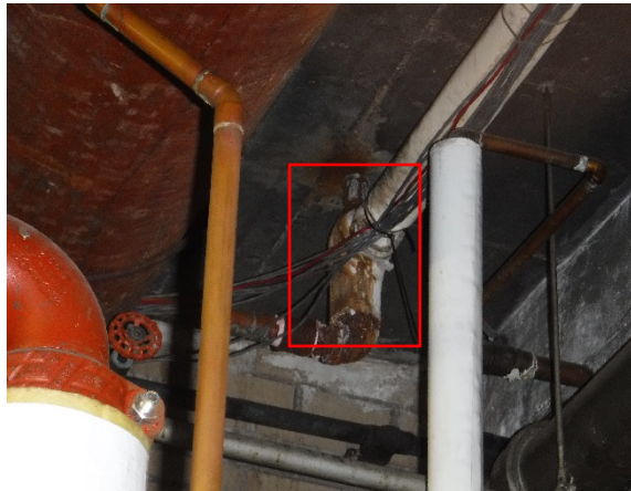
Photo 34: Example Photo of Remaining ACM Piping Insulation – Mechanical Room.
