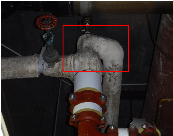
Photo 33: Example Photo of Remaining ACM Piping Insulation – Mechanical Room.
