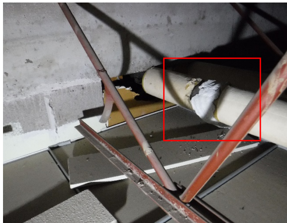
Photo 30: Example Photo of Poor Condition, Unwrapped ACM Piping Insulation, Fitting – Room 104, Ceiling Cavity.
