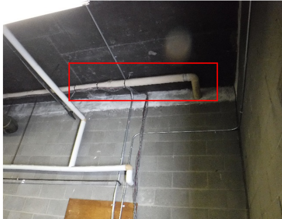
Photo 32: Example Photo of Remaining ACM Piping Insulation – Mechanical Room.
