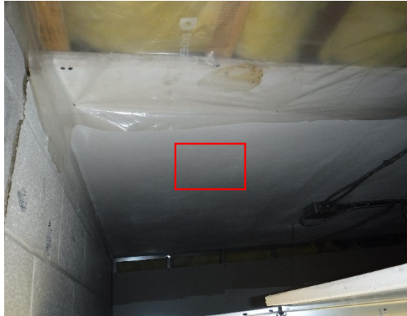
Photo 8: Photo of sample AS-15, Room 127, Ceiling – Texture Coating, 1% Chrysotile Asbestos.
