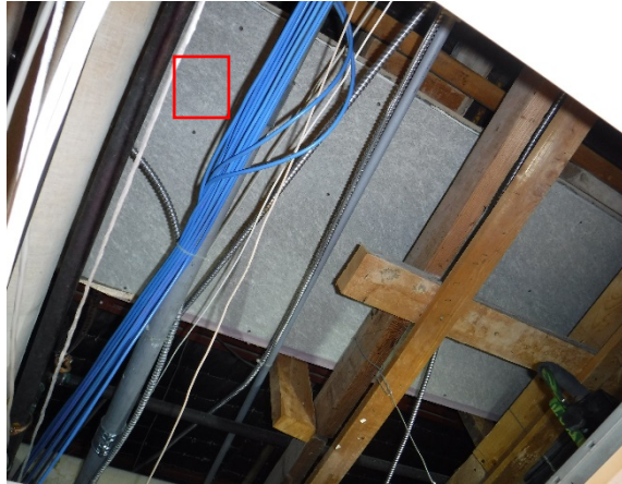
Photo 20: Photo of transite panel found in Hallway (SW), Ceiling Cavity – Visually similar to EXT-AS-01, 13.6% Chrysotile Asbestos.
