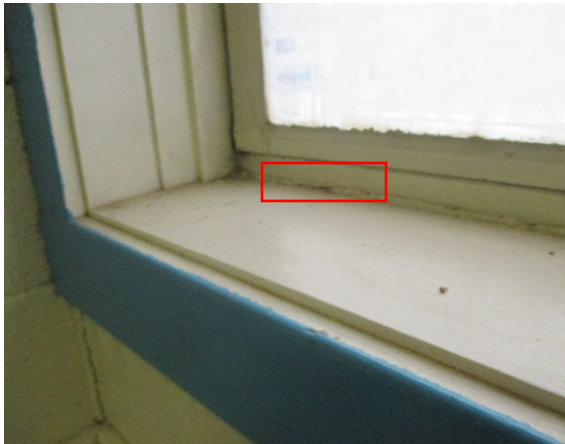
Photo 9: Photo of sample AS-19, Men's Washroom, Window – Caulking Material, 2% Chrysotile Asbestos.
